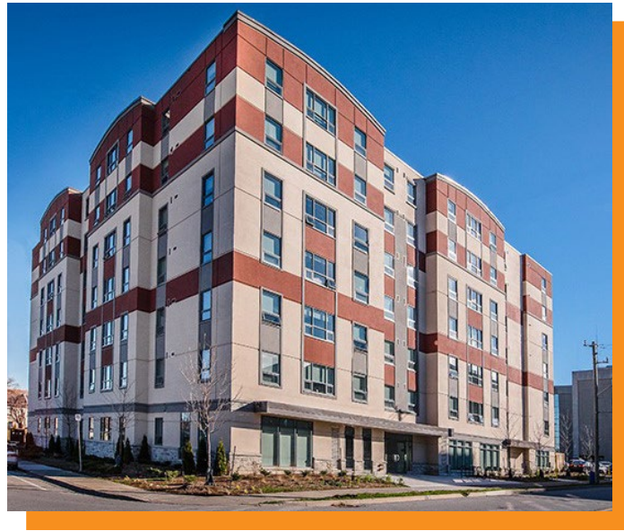
This 7-story building was built ahead of schedule & below budget by utilizing the RIC system
