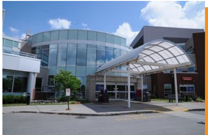
Construction of this important new hospital addition was completed rapidly using the Geopier GP3®
