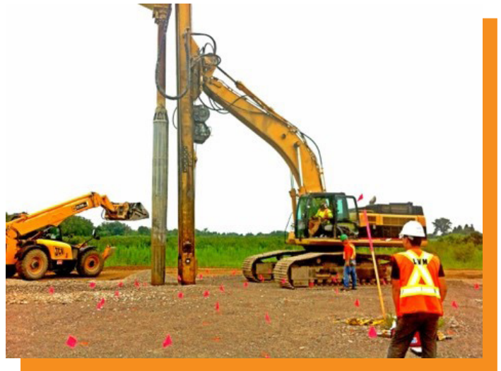
Installation of the Armorpack® system at Oxley Wind
