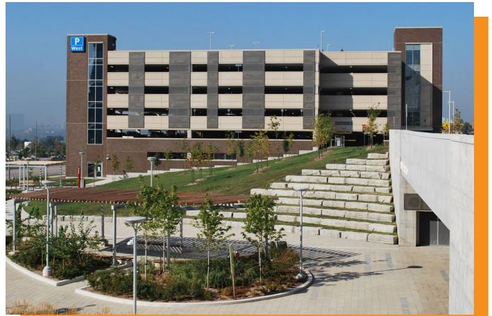
Humber River Hospital received LEED® Gold certification due in part by utilizing the Geopier GP3® system
