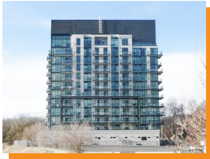
The Grand Condominium rests on high capacity spread footings on ground improvement at the basement level in soils that had SPT-N Values of 0 to 2 for over 30 feet in depth
