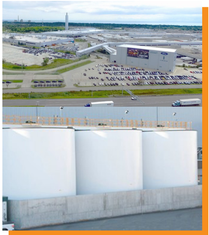
These three very large tanks are supported by Geopier® elements resulting in considerable cost savings when compared to dig/replace
