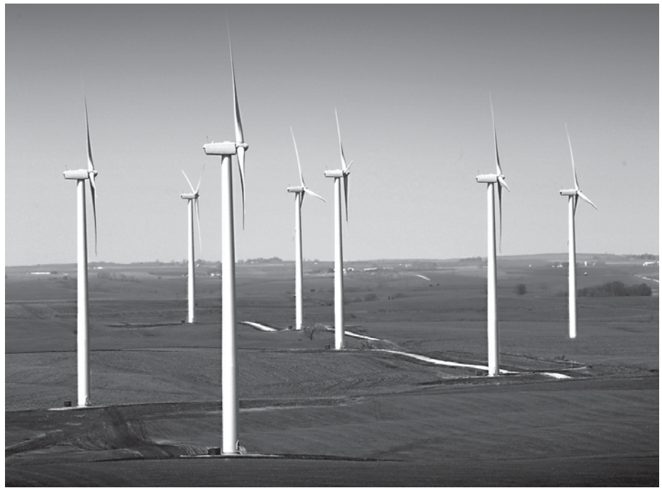
Environmentally friendly foundation technology was used at the Victory Wind Farm, shown here.
