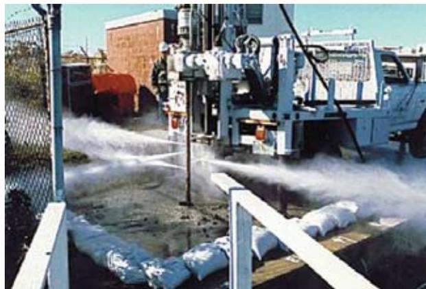
Figure 4. Jet grouting. Photo courtesy of Earth Tech.
