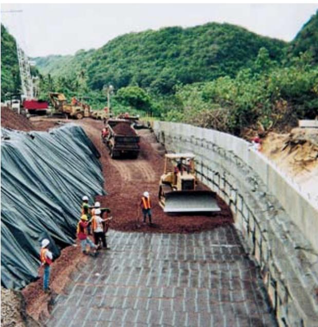
Figure 2. Mechanically Stabilized Earth (MSE) walls. Photo courtesy of The Tensar Corporation.
