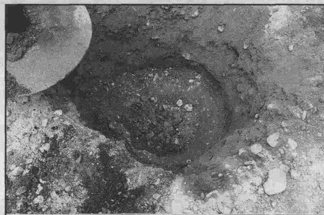
Completed Geopier element
