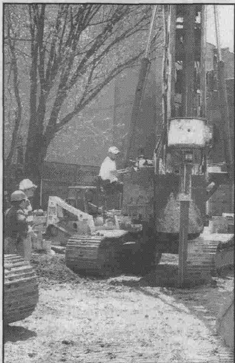
Drilling piers on a tight site
