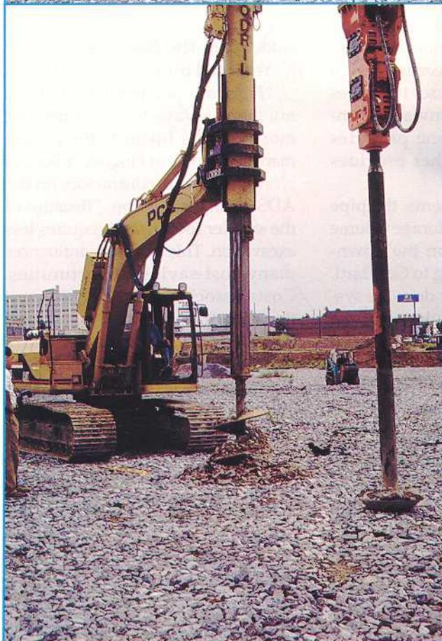
Auger mounted on an excavator bores hole for Geopier installation.
