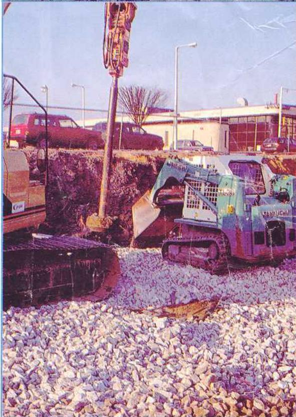
Tampers attached to hydraulic breakers on either an excavator or a skid-steer loader are used to compact the lifts of aggregate that make up the Geopier.
