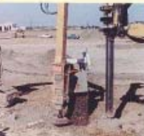
DRIVING Rammed piers system cut costs and time.
