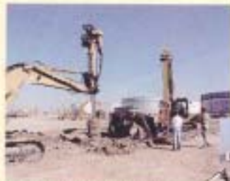
DRIVING Rammed piers system cut costs and time.
