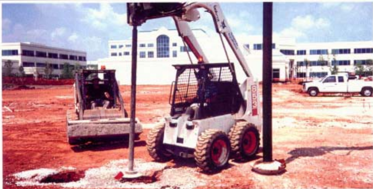
GEOPIERS: Soil reinforcement technology reduces settlement, offers time and cost advantages.
